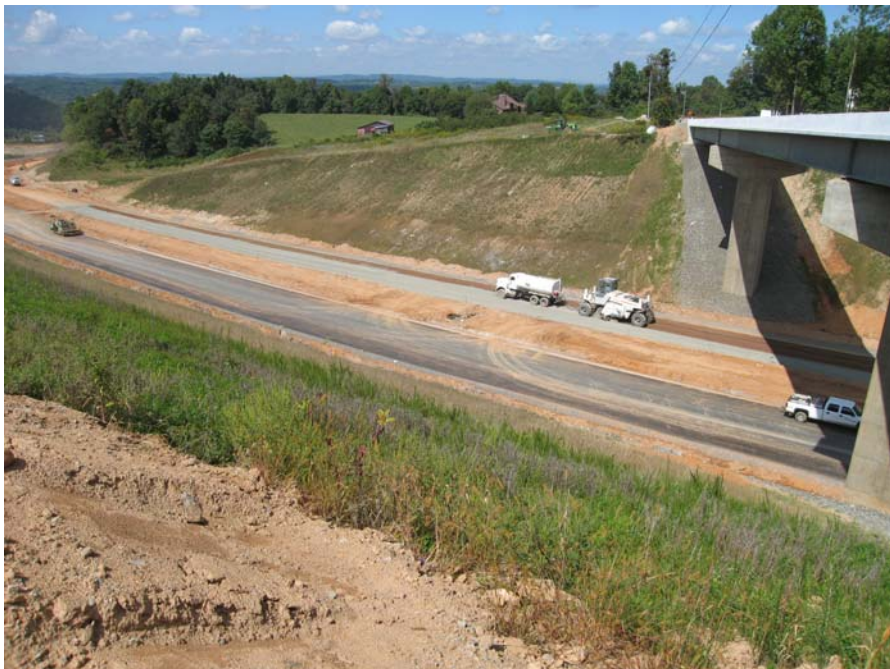
Image 6 - Area 3, Subgrade Cement Stabilization below Howlett St. Bridge (9-14-09)
