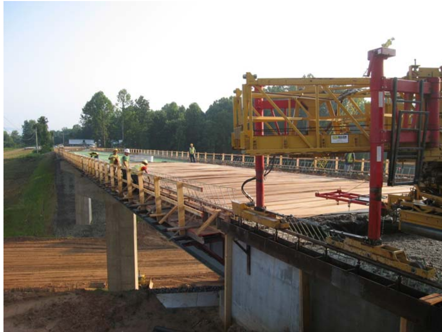
Image 7 - Area 4, B615 Howlett St. Bridge deck concrete (7-10-09)
