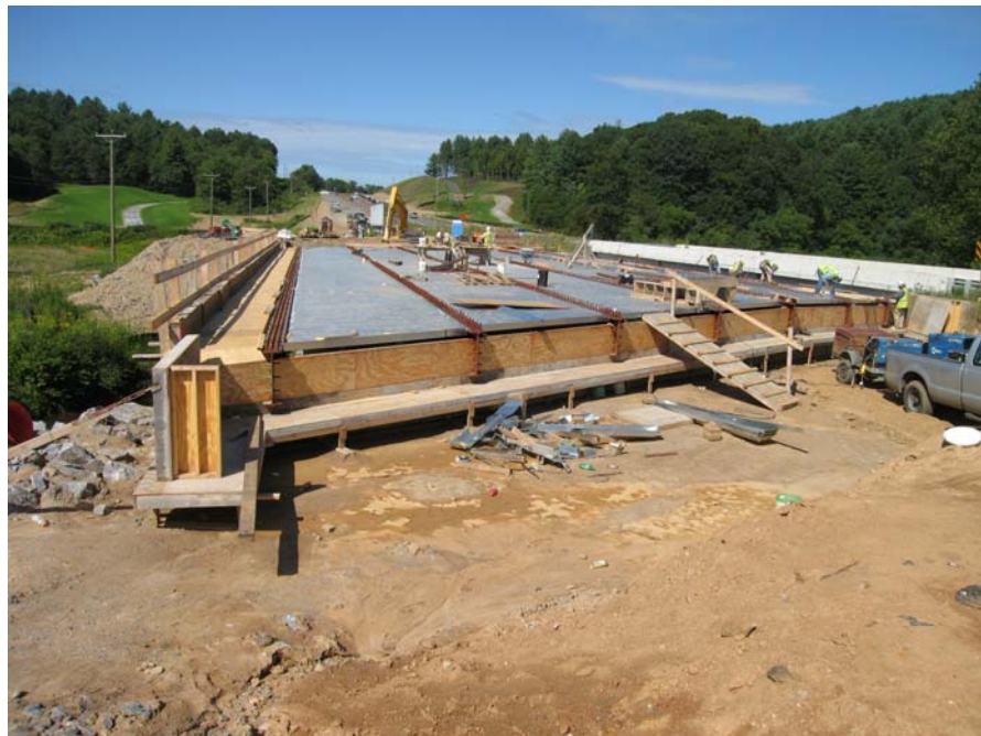
Image 2 - Area 2, B617 deck pan installation (8-17-09)
