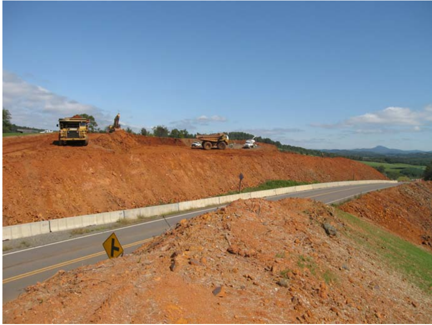
Image 9 - Area 6, Ramp I excavation (9-30-09)
