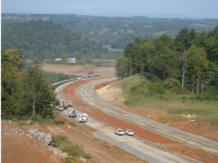
Image 5 - Area 3, Base asphalt east bound, and base CTA west bound (9-28-09)
