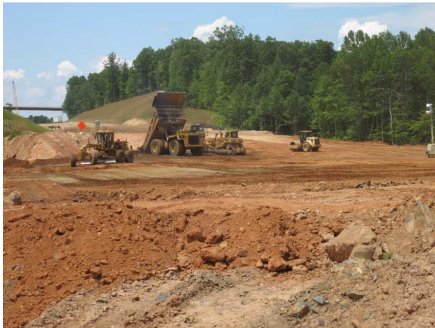
Image 8 - Area 4, Fill 5 work, this has since completed (7-13-09)
