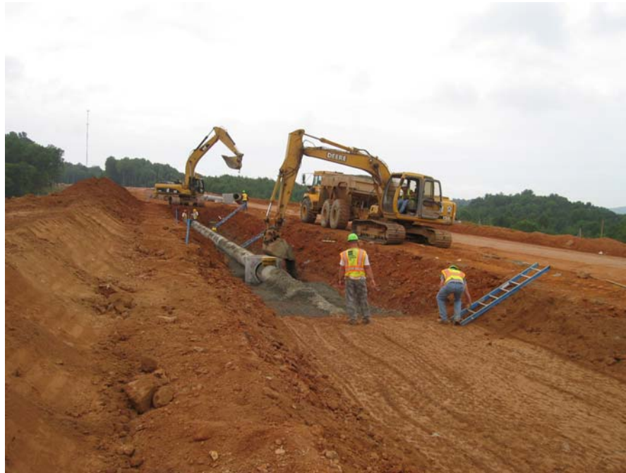
Image 3 - Area 3, Median pipe work Mainline Bypass (7-16-09)
