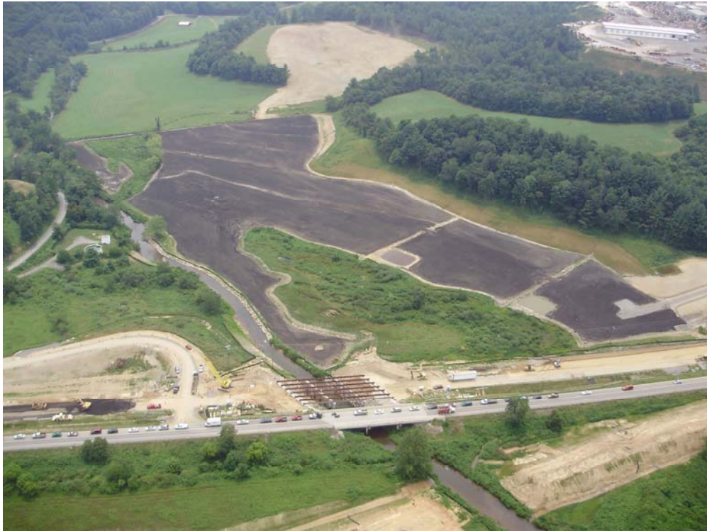
Image 1 - Area 1, Webb Wetland Mitigation Site (7-22-09)
