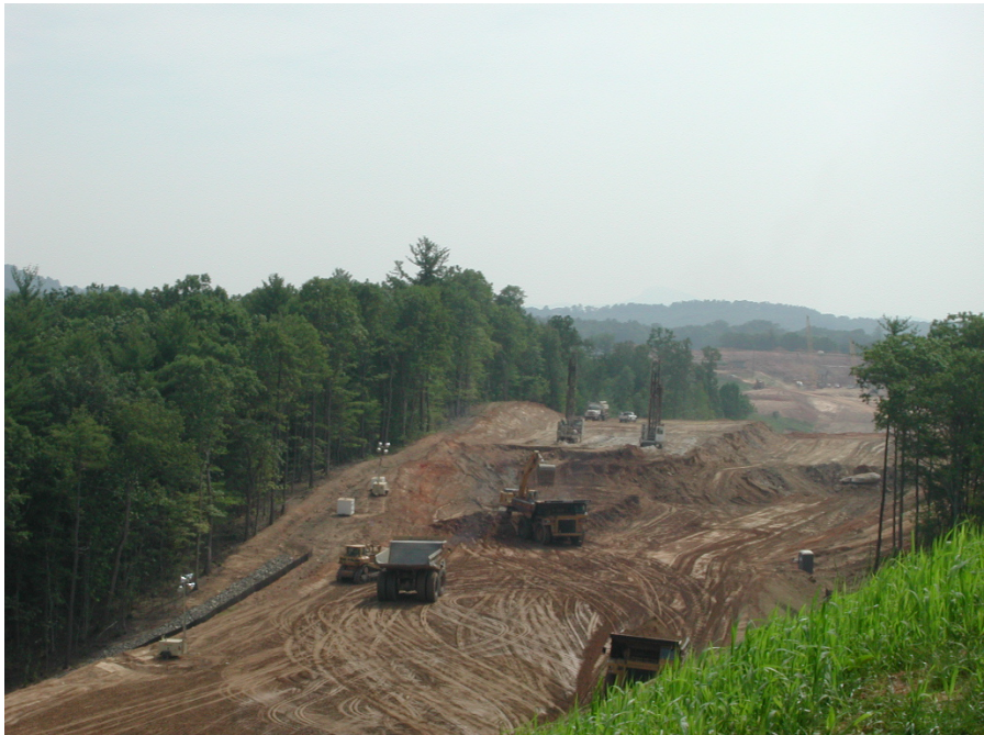
Image 4 - Work Area 4, Cut between Howlett and Rt. 52, Station 120+00 to 125+00 (7-22-08)
