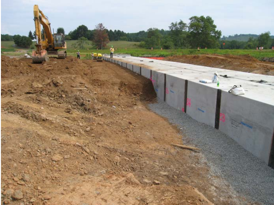
Image 5 - Work Area 5, Box Culvert 24-1 (8-25-08)
