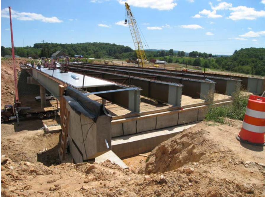
Image 3 - Work Area 4, B-614 steel and deck (8-11-08)
