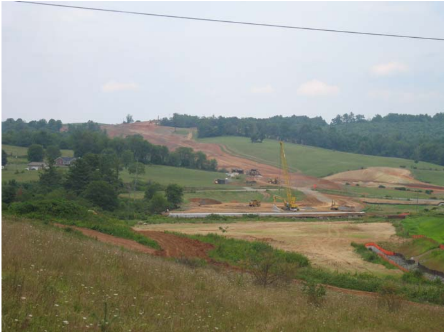
Image 6 - Work Area 5+6, Box 24-1 near with crane, Mass cut Station 155+75 to 169+50 background (9-4-08)
