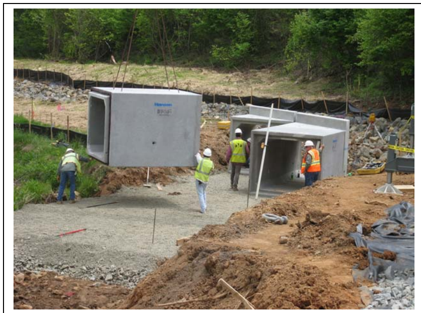
Image 6 - Work Area 6, Phase I of Box Culvert 34-17 (5-14-09)
