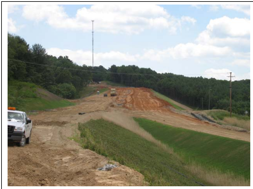
Image 2 - Work Area 3, Mainline Bypass Box+Balance (6-30-09)
