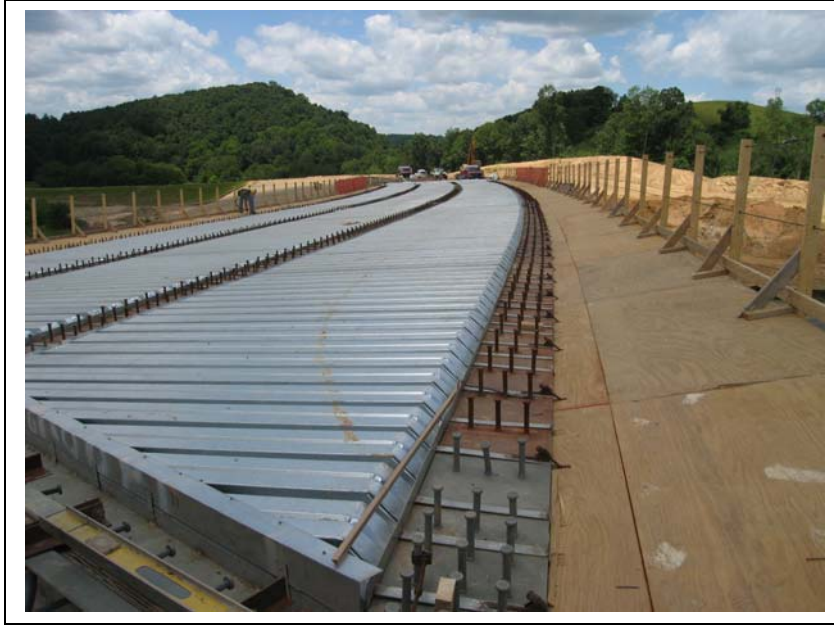
Image 1 - Work Area 2, B-616 Deck Pans (6-30-09)
