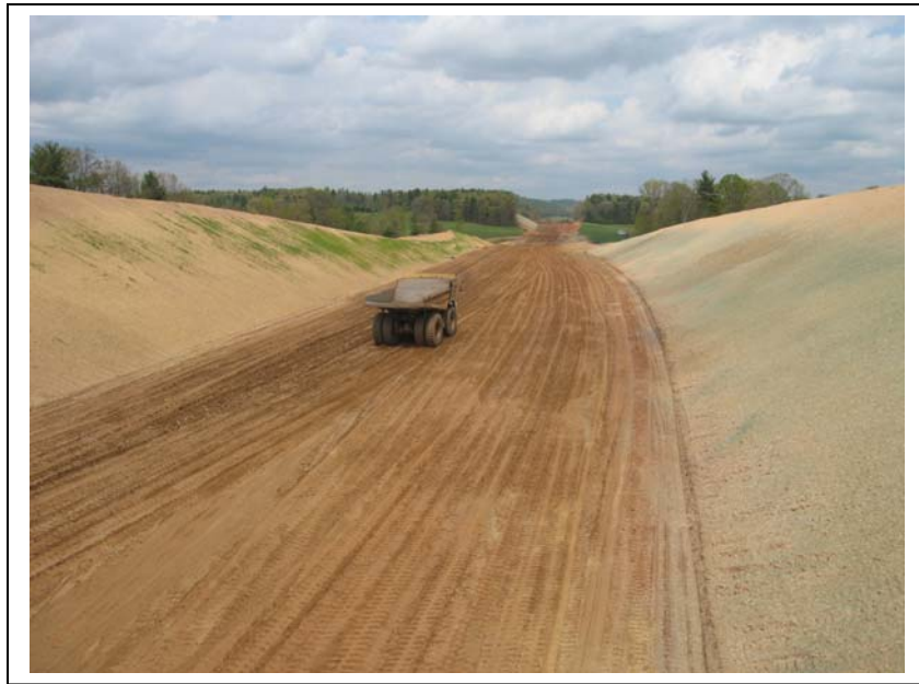
Image 4 - Work Area 5, Mainline Bypass Sta. 132 look East (4-29-09)
