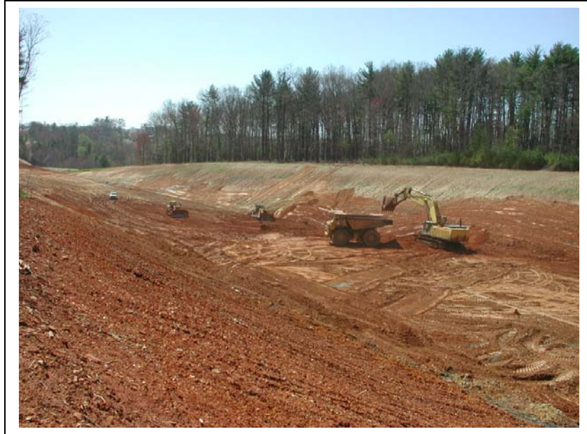
Image 5 - Work Area 5, Mass Excavation at Sta. 140 (4-23-09)
