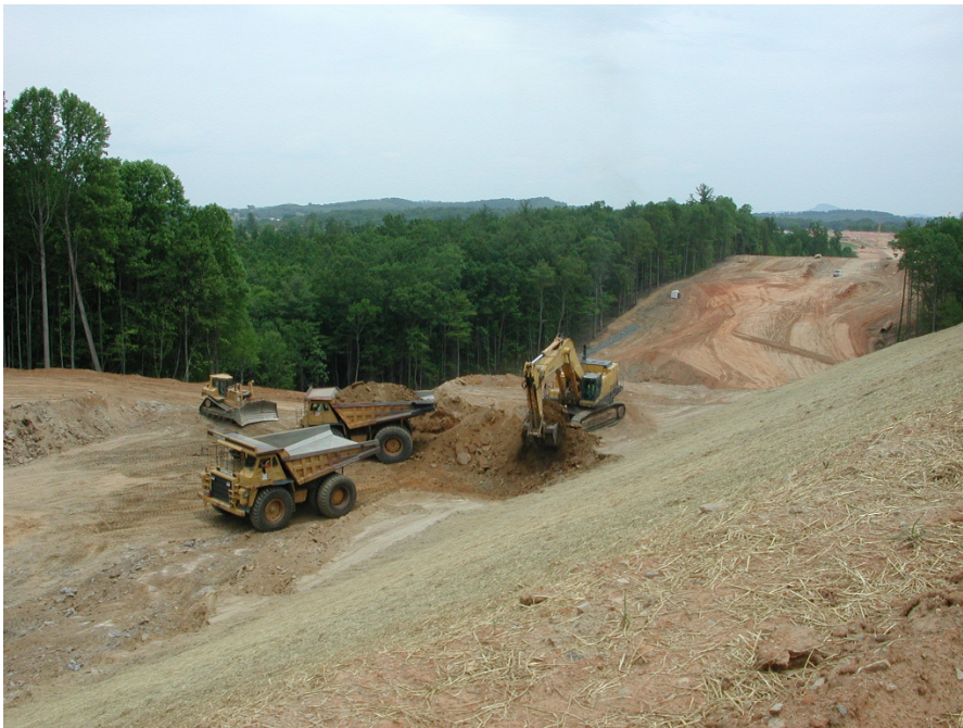
Image 2 – Work Area 3, Kanawha Stone Cut at Howlett Street (6-20-08)
