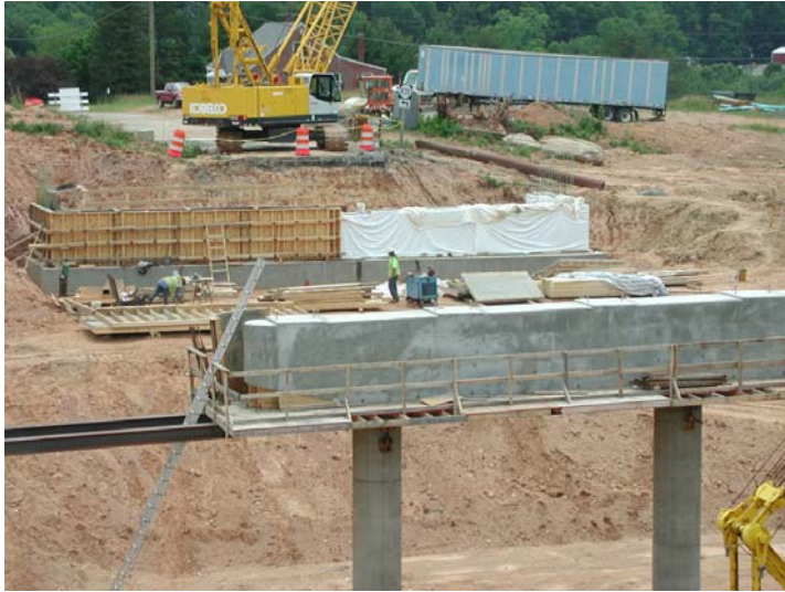
Image 5 – Work Area 4, B-614 Pier and Abutment A (6-20-08)
