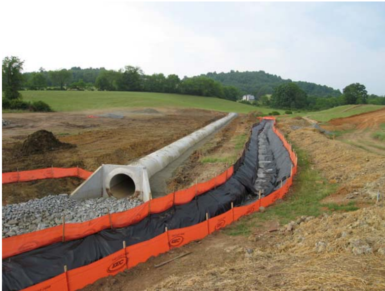
Image 6 – Work Area 5, Deep Pipe #25-7 (6-13-08)
