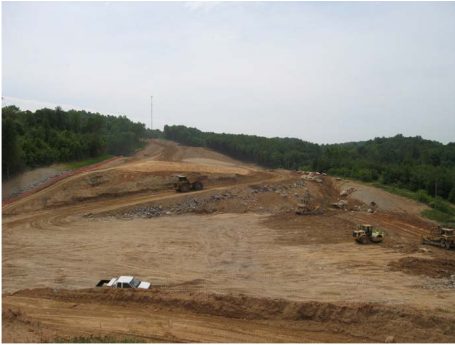
Image 3 – Work Area 3, Kanawha Stone Fill at Deep Pipe #9-8 (6-3-08)
