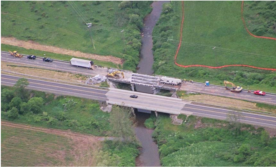
Image 1 – Work Area 2, B-617 Demolition (5-30-08)
