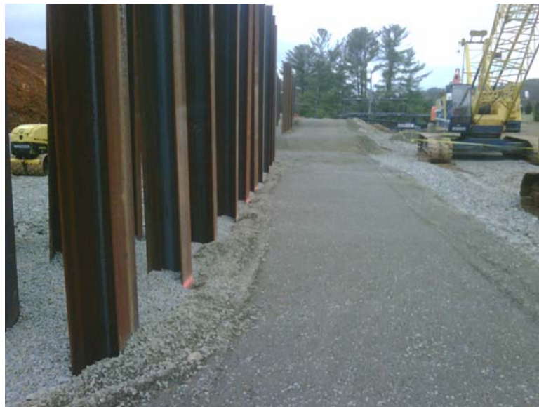
Image 4 - B612+613 aggregate base for MSE leveling pad, west abutment, 3/26/10
