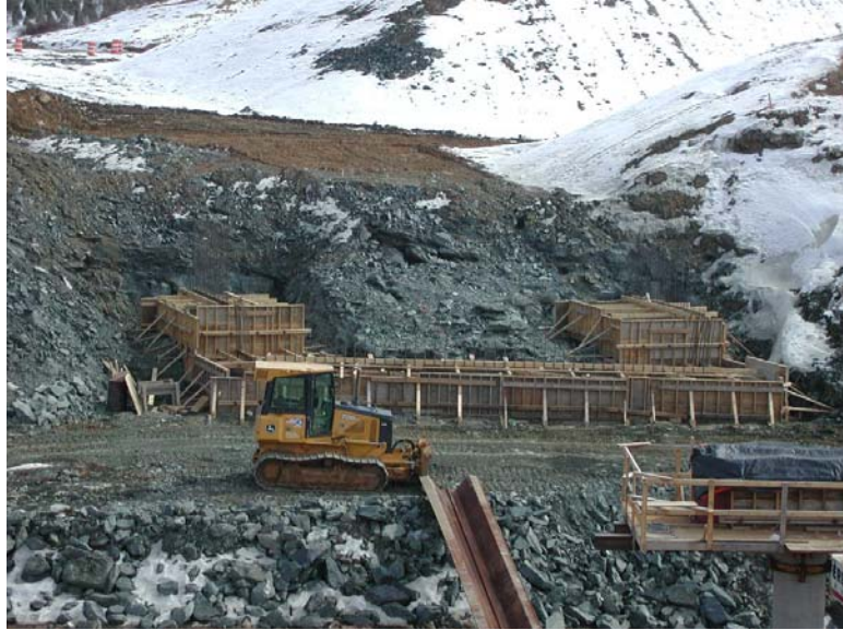
Image 7 - B611 looking south, Abutment B 3/1/10
