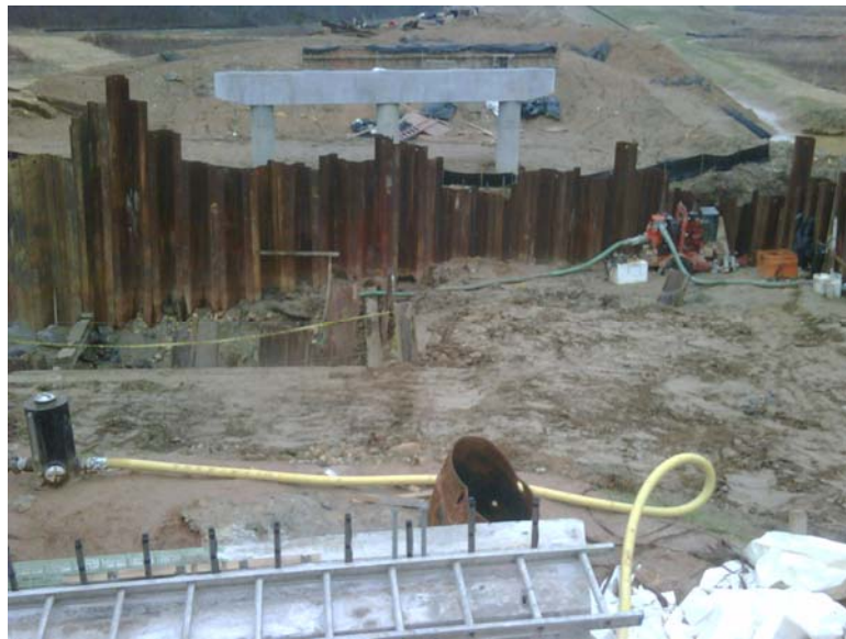
Image 2 - B618 west cofferdam looking east, 3/26/10
