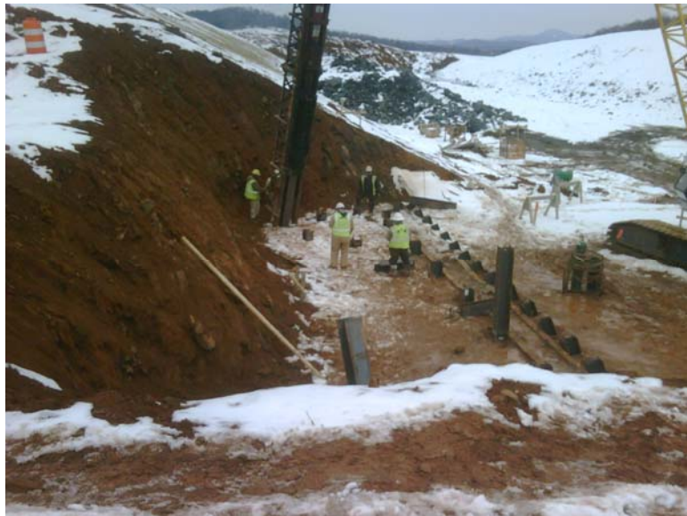
Image 8 - B611 Abutment A driving h-pile, 2/4/10
