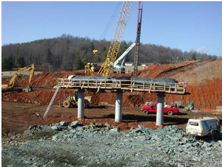
Image 6 - B611 looking north, pier and Abutment A h-pile, 1/28/10
