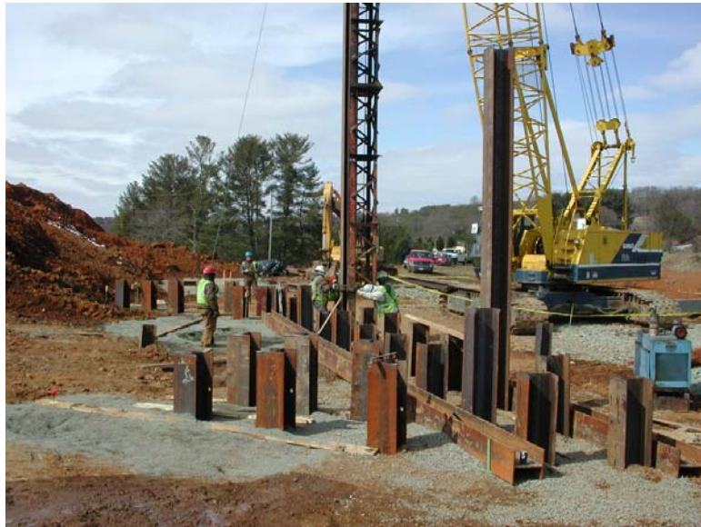
Image 3 - B612+613 west side h-pile, 3/1/10
