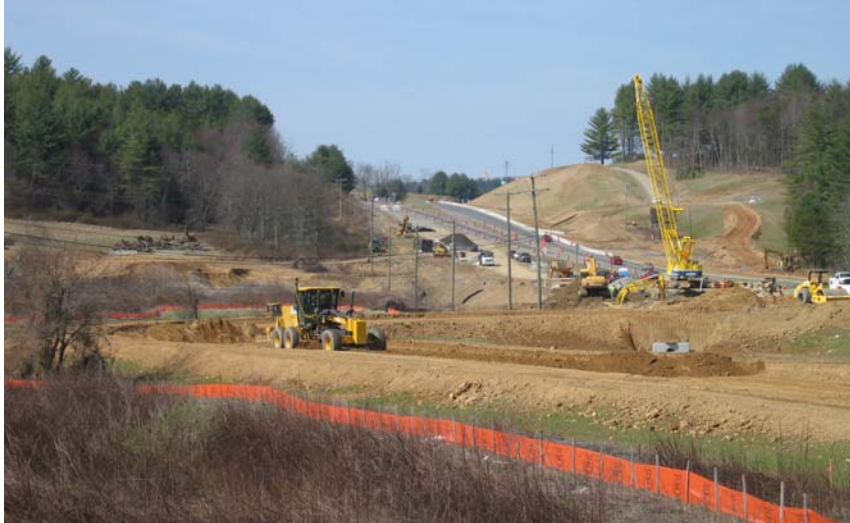
Image 3 - Area 2, fine grading Gardner's Mill Road with GPS Grader (3-23-09)
