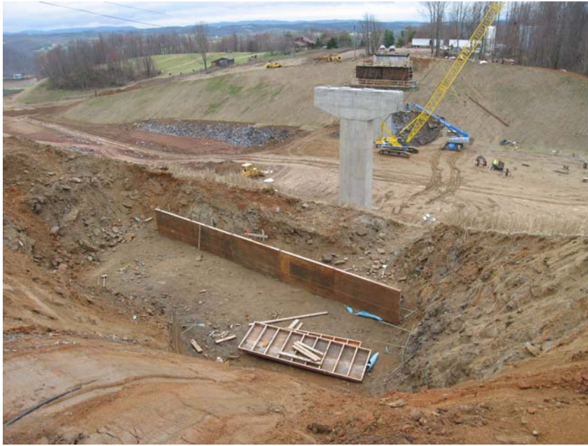
Image 5 – Area 4, B-615 Howlett St. looking N, Abutment B and Pier #2 near (3-27-09)
