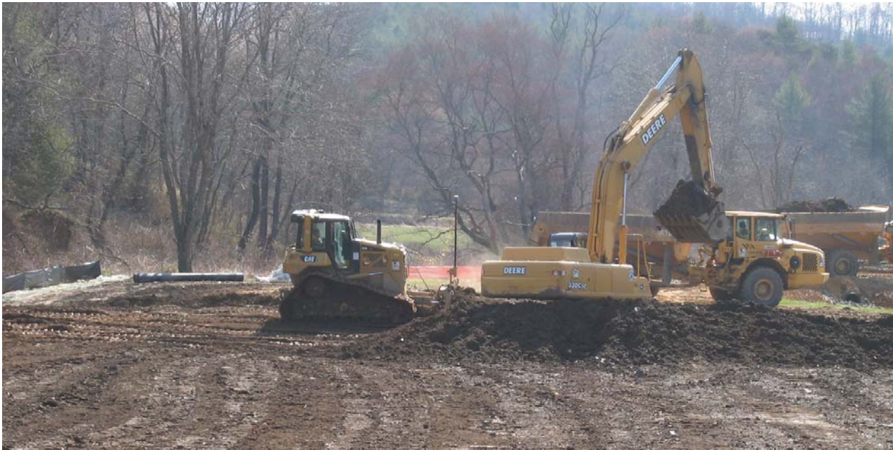
Image 1 - Area 1 Webb Wetlands, grading cell #1 with GPS D6 bulldozer (3-23-2009)
