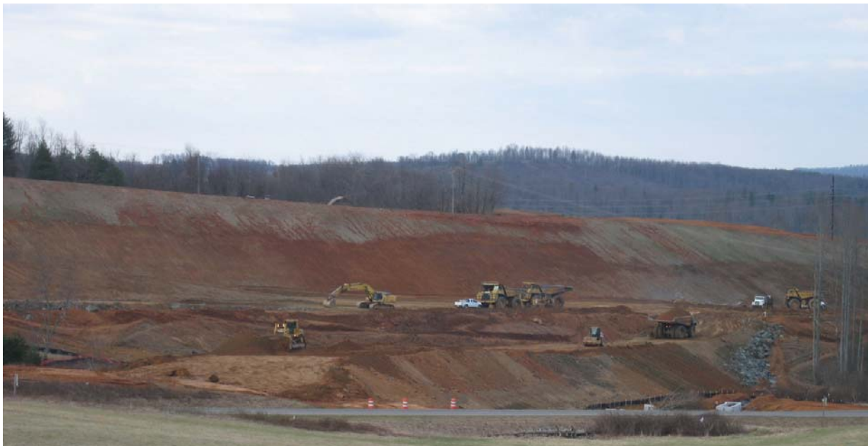
Image 6 - Area 6, Fill at Ramp L, looking from Rt. 669 (3-23-09)
