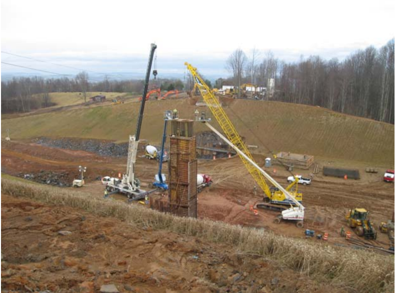
Image 4 - Area 3/4, South Pier Column Concrete Placement B-615 Howlett St. (12/18/08)
