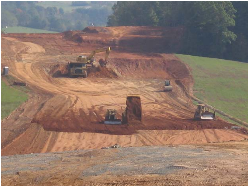
Image 6 - Area 5, Mass Excavation near Station 140+00 (10/6/08)
