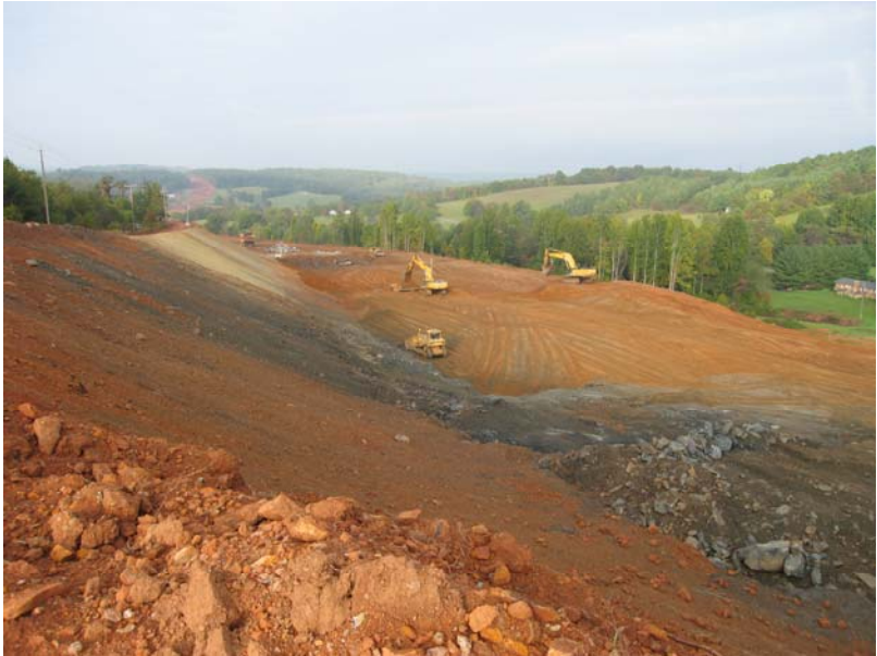
Image 8 - Area 6, Cut 6 looking West near station 162+00 (10/1/08)
