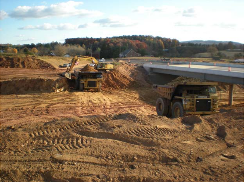
Image 5 - Area 5, Mass Excavation at Rt. 52, B-614 open to traffic (11/5/08)
