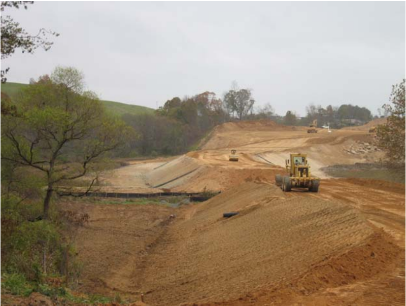
Image 3 - Area 2, Bridge B-618 approach fills Rt. 58 Bypass WBL (10/24/08)
