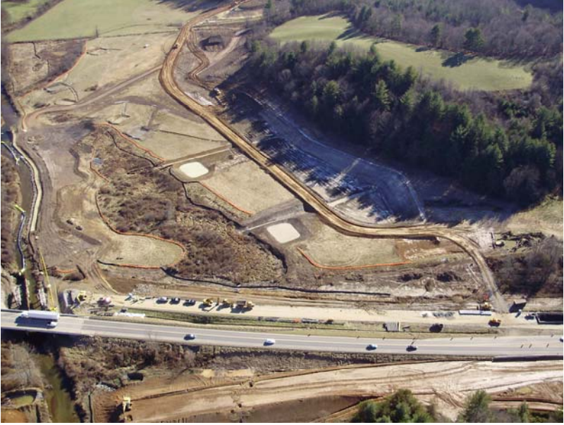
Image 1 - Area 1, Webb Wetlands Mitigation Construction (12/3/08)
