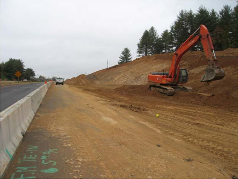
Image 2 - Area 2, Widening of existing Rt. 58/221 WBL (10/24/08)
